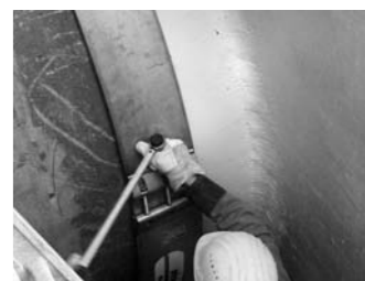
The pressure required to ensure a secure seal is built up by tightening the lock parts.
